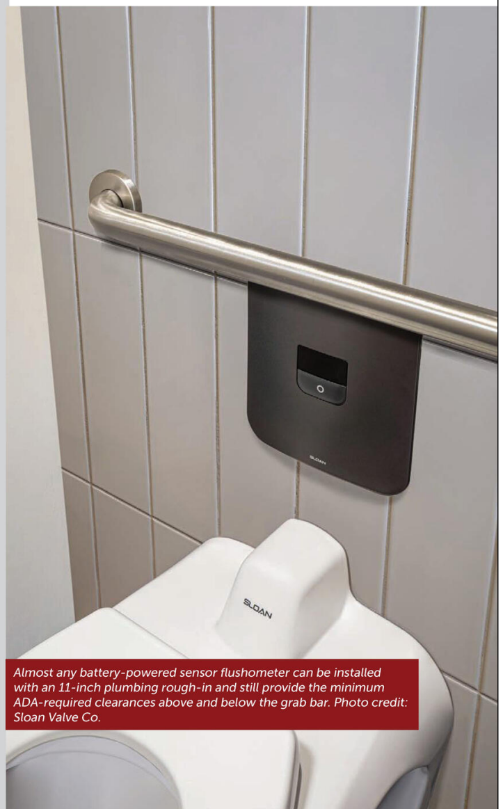
In the commercial restroom, the flushometer is the most accepted and reliable means for water closet and urinal functionality. Photo credit: Sloan Valve Co.
